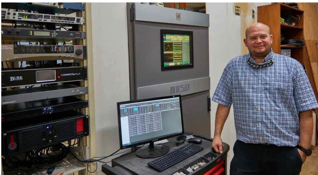
Aaron Farnham of Bonneville's KSL with the Orban XPN-AM user interface on the monitor and the hardware in the rack to the left.
