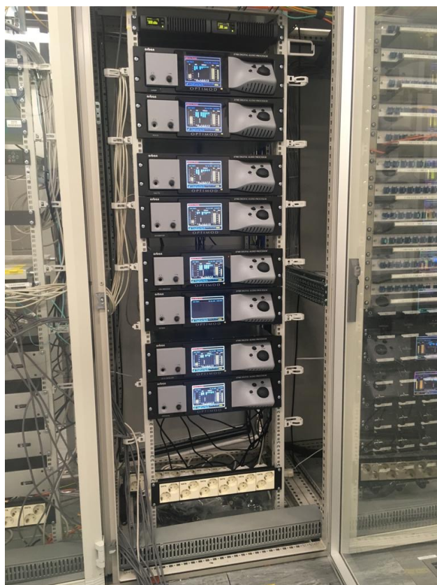
Rack with OPTIMOD 8700i Audio Processors
